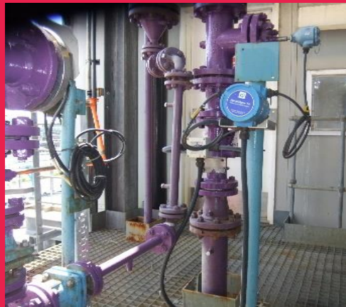
DensicheckTX in service at Ineos, Runcorn
